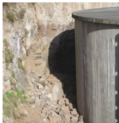
Figure 8 – McCormacks Bay reservoirs – access road damage and rock fall around reservoirs
