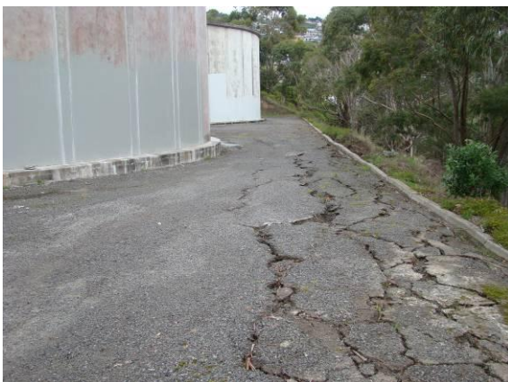
Figure 8 – McCormacks Bay reservoirs – access road damage and rock fall around reservoirs
