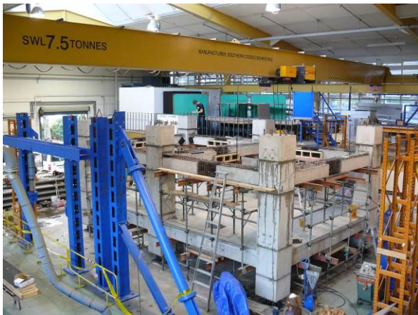
(c) Second floor precast components being grouted
