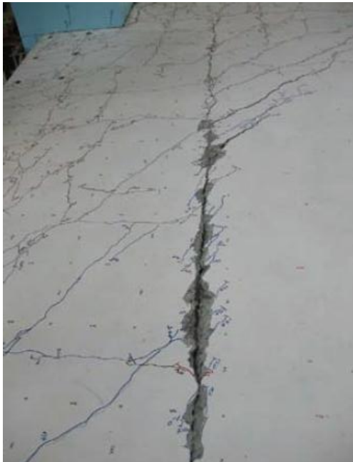
(d) Timber infill cracks, approximately 8mm (Lindsay 2004).
