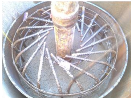
Figure 6: Concreting using Tremie pipe
