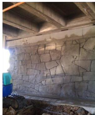
Figure 12: Final product of the shotcrete wall and footing
