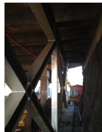
Figure 13: Completed auxiliary support
