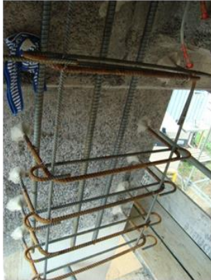
Figure 14: Bolster reinforcement
