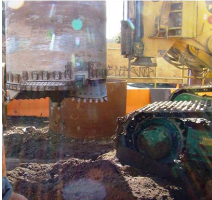
Figure 3: Bauerer rig in action with the rotary barrel
