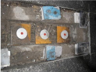
Figure 15: Anchors plate with threaded inserts in pockets prior to grouting
