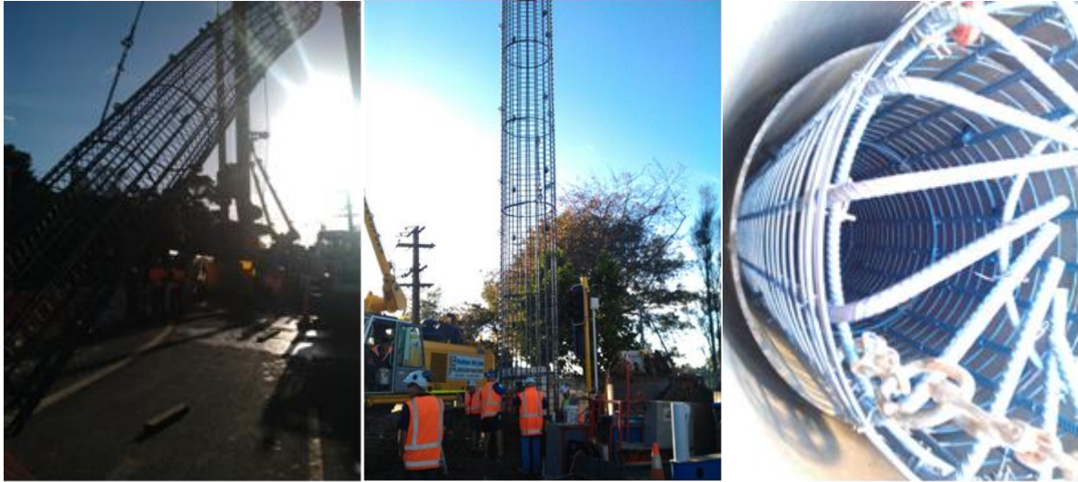
Figure 5: Lifting and lowering of pile cage into bored hole
