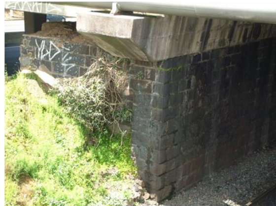
Figure 10: Existing wingwall to be demolished
