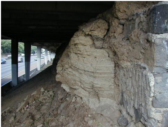
Figure 9: Soil leaning against the basalt wall prior to excavation
