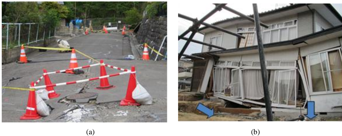
Figure 9: Slope failure in Oritate 5-chome: (a) damaged road; and (b) deformed house.
