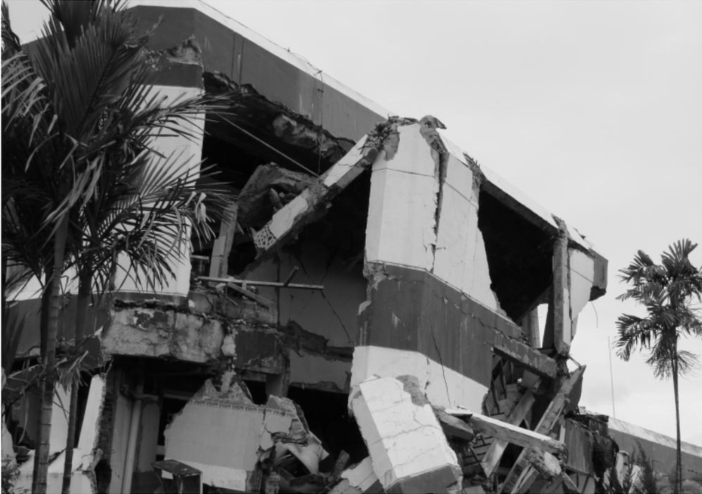
Figure 2. Damage to the main hospital in Padang, Indonesia, after the 30 September 2009 Western Sumatra (M=7.6) earthquake
