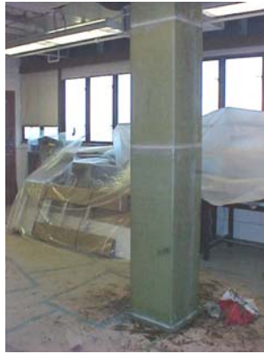
Figure 5. The Tyfo ® SEH Composite System installed over a square column.
