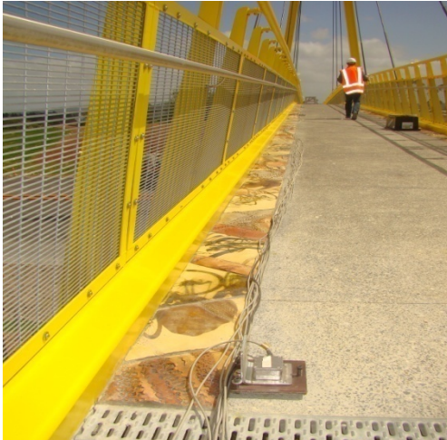
Figure 5. Accelerometers placed on the bridge to measure structural response
