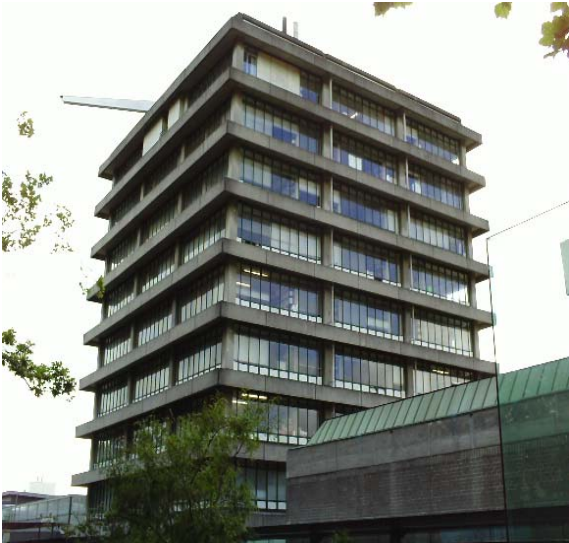
Figure 1 South and west face of the engineering building
