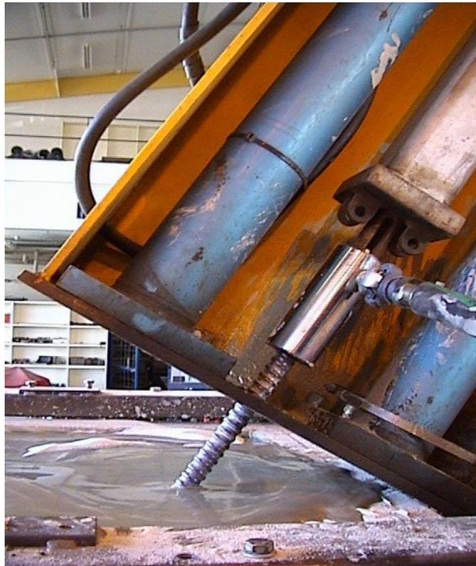
Figure 7. Installation of inclined micropiles.
