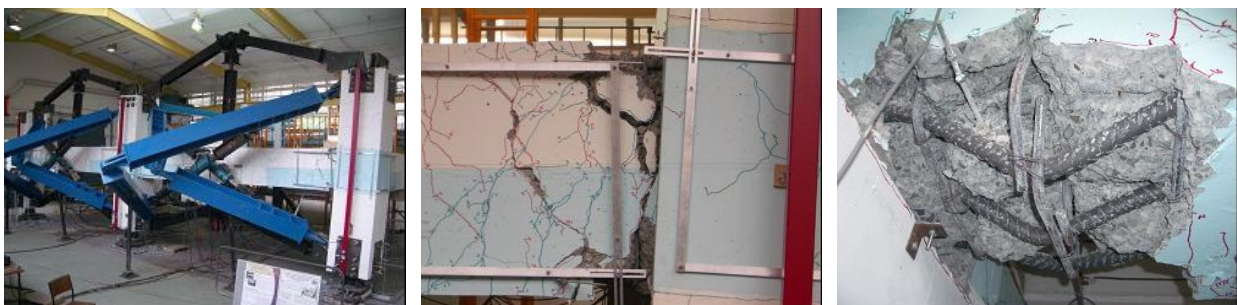
(a) Super-assembly specimen at +5% drift. (b) Damage of the southeast plastic hinge at +5% drift. (c) Longitudinal beam bar buckling.
