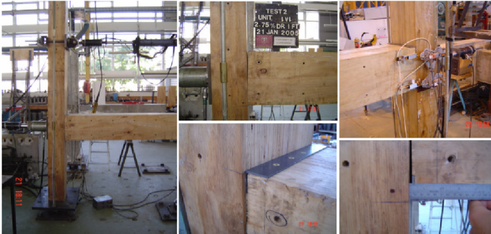
Figure 8. Unbonded post-tensioned solution: performance of the specimen ( 0.6 f_{py} ) at drift level of 2.75%.
