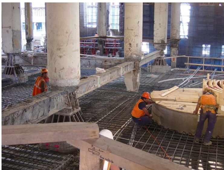
Figure 4 : Lowering the Ground Floor
