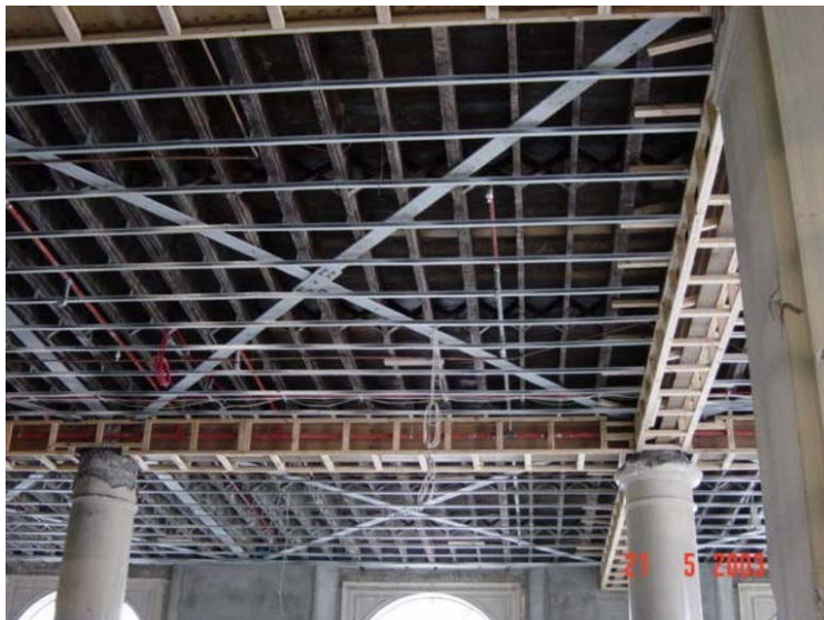
Figure 3 : Steel Floor Diaphragm
