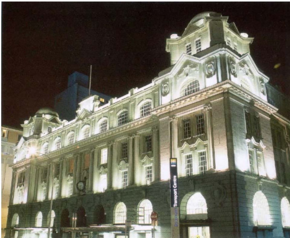
Figure 1 : Front of Building
