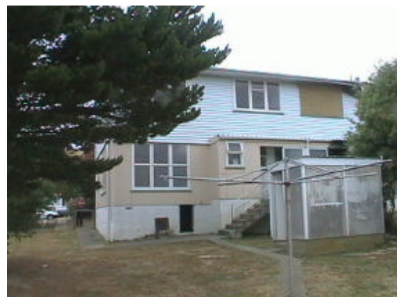
Figure 6: 1960s two-storey wood-framed duplex unit (central wall at both levels was evaluated)
