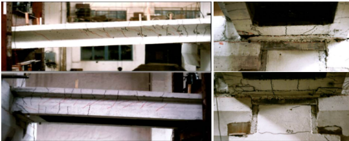
Figure 11 Details of the tested joint at the Damage Control Limit State
