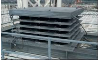
Figure 9. Tuned mass damper
