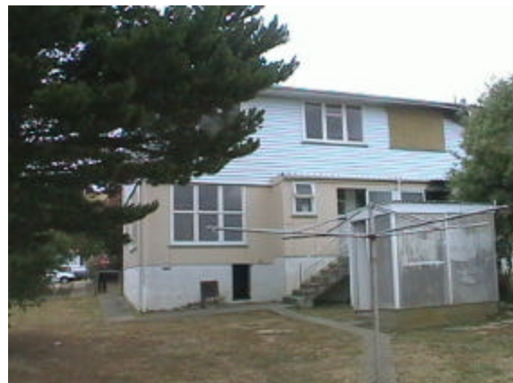
Figure 6: 1960s two-storey wood-framed duplex unit (central wall at both levels was evaluated)
