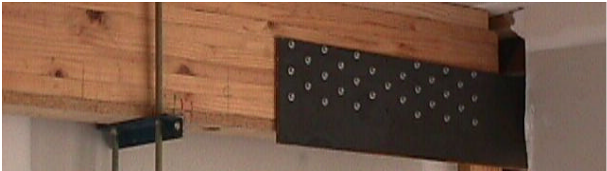
(b) Connection to timber loading beams
