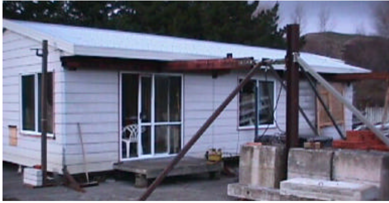
(a) General view of test in progress
