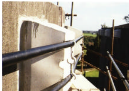
Figure 11: Close up of spacer block for roof strengthening and stressing cable make up
