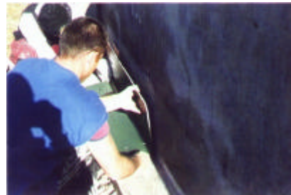
Figure 6: Installation of base L-shaped steel seismic shear coupons
