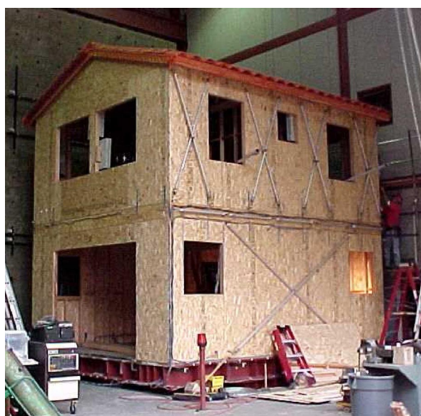
View of Building from NorthWest
